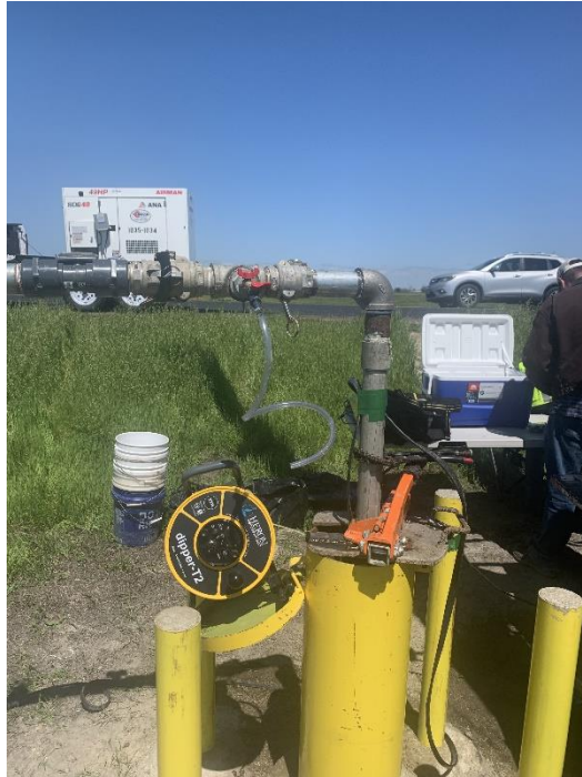
Photograph 9. Pump and Other Equipment Installed Within TW-1 for Development
