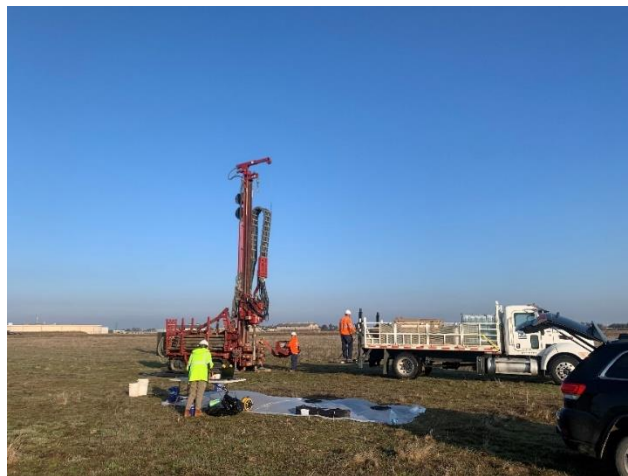
Photograph 2. Sonic Drill Rig Used for Completion of Soil Borings
